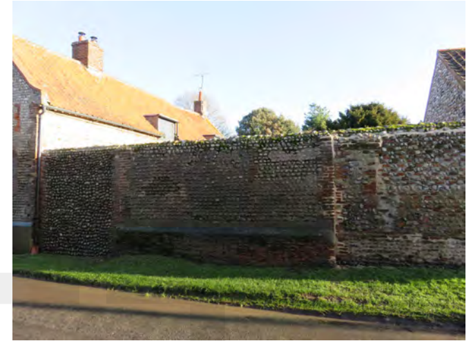
Grade II listed wall to Green Farm
