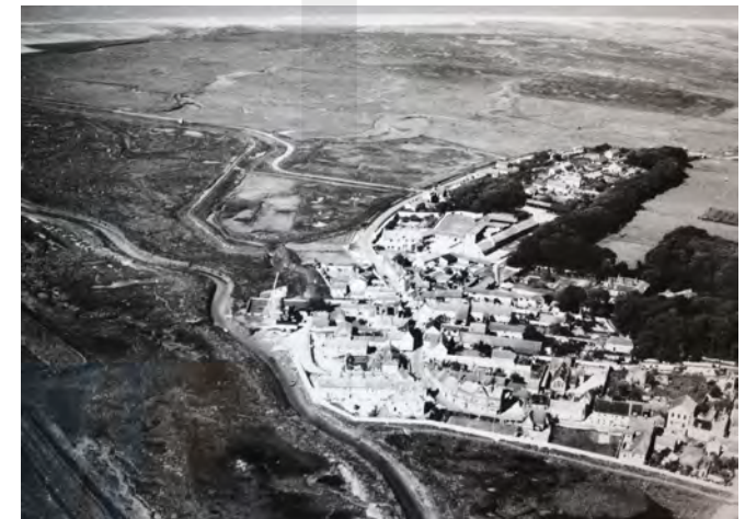
Aerial view of the north of Cley looking east, c.1964 (Image courtesy of Norfolk Heritage Centre, Norfolk and Norwich Millennium Library: C/CLE 12092y)
