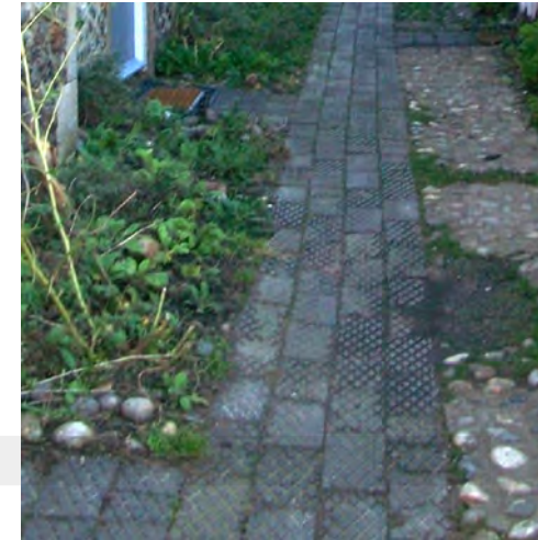
Detail of the paving to the footpaths
