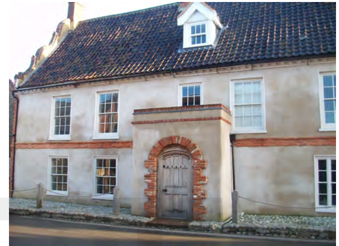
Sunbeams, an example of a high-status house employing a vernacular style, with prominent Dutch gables.
