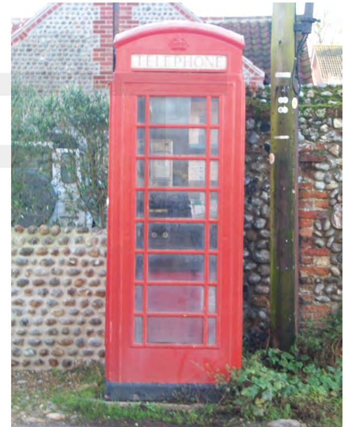
K6 Telephone box, Grade II Listed
